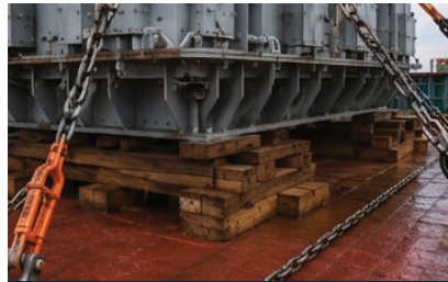
Wooden Blocking & Cribbing
